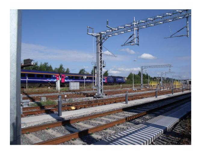
Electrification reaches Wales! The view outside of Swansea station on the 9<sup>th</sup> September with the masts and booms in place above the tracks leading to the new Hitachi depot for the Super Express trains. In the background an Inter City125, which will be replaced by the new trains, is setting out on its 190 mile journey to London. (photo: PK)
