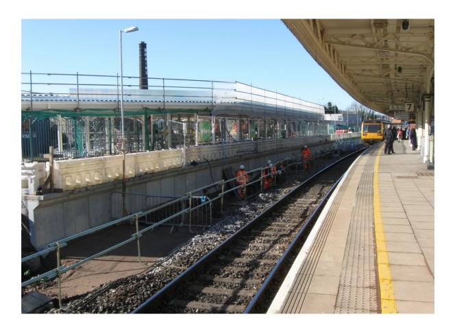
ON 17<sup>th</sup> February 2015 work is progressing to prepare the track bed at the new Platform 8 at Cardiff Central. On the left of the picture, the new southern entrance to the station is under construction; this is expected to open this summer. (photo: Julian Langston)
